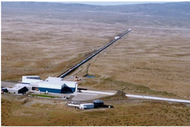
FIG. 2: An aerial view of the LIGO observatory at Hanford, Washington is shown above. Evacuated beam tubes extend from the building, in which lasers and optics are kept. The full length of one H1 arm is shown; the arms of the H1 detector each extend 4 km. They are perpendicular to each other and enclosed in concrete. The 2km-long H2 detector also occupies the beam tubes. That detector was not in operation during the LIGO S6 run. Adapted from [1].
