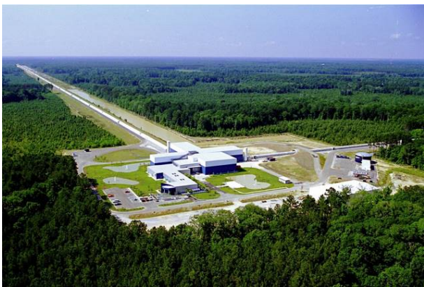
FIG. 3: An aerial view of the LIGO observatory at Livingston, Louisiana is shown above. As in the Hanford observatory, the beam tubes are at right angles to each other and extend 4 km in each direction. Adapted from [1].
