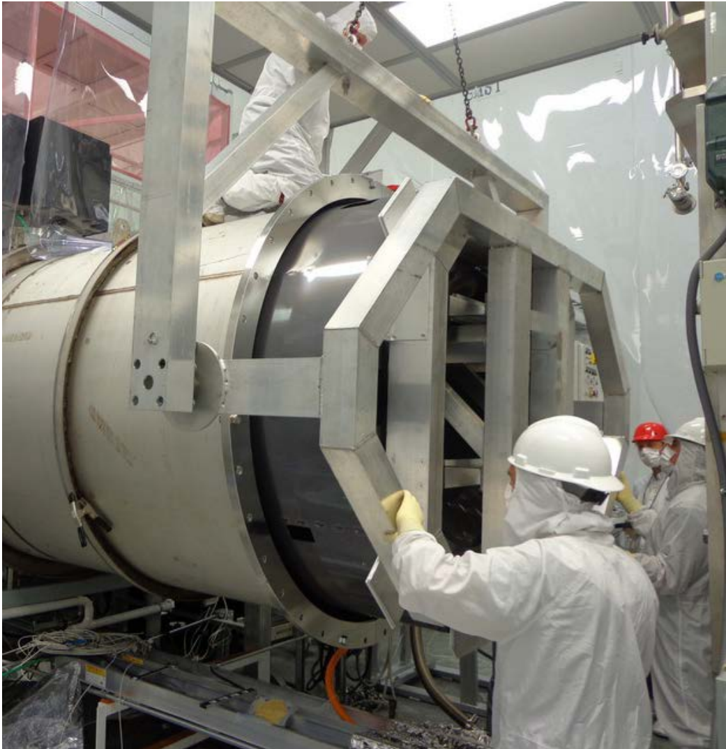
Figure 35: Baffle insertion into Adapter
