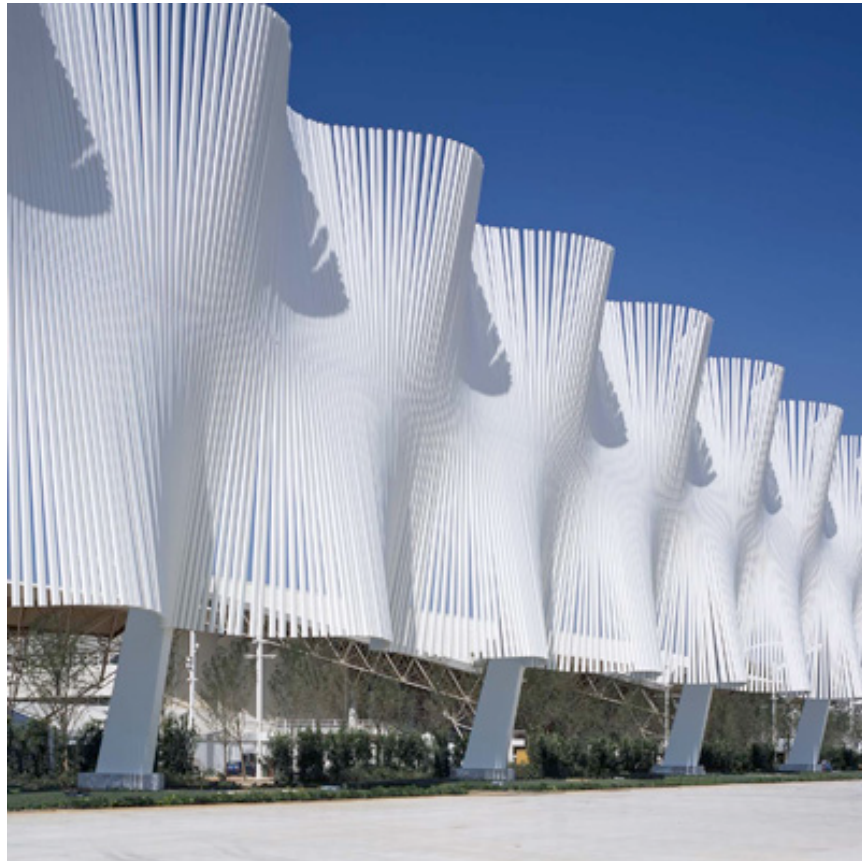
Figure 4: A (static) architectural frontispiece at the Athens Olympics sports complex, suggesting the scale and visual impact of the planned SEC façade. (Santiago Calatropa, 2004)
