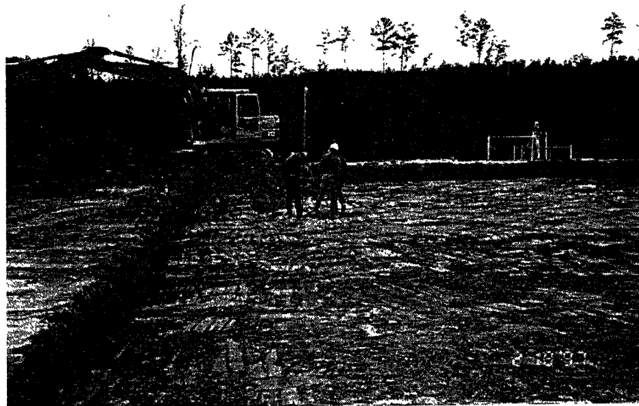
FIGURE 18. Excavation for the Foundation for the End Station on Southeast Arm at the Livingston Site.
