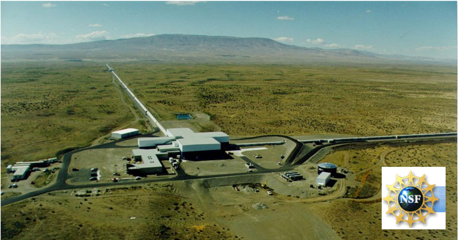
Two separate interferometers (4 km and 2 km arms) coexist in the beam tubes
