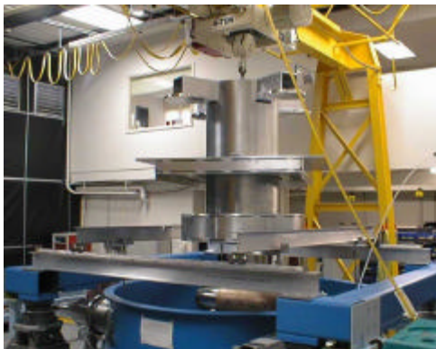
Figure 26. Downtube being Hoisted
