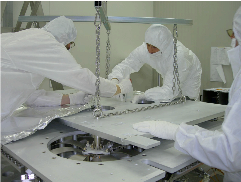
Optical table support plate being installed. It sits on a modified kinematic mount on the four filter key-stones. The optical bench slides over and bolts on this plate
