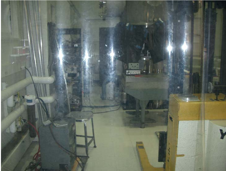
Figure 16 Route position 5. From within portable clean room (which will be removed).
