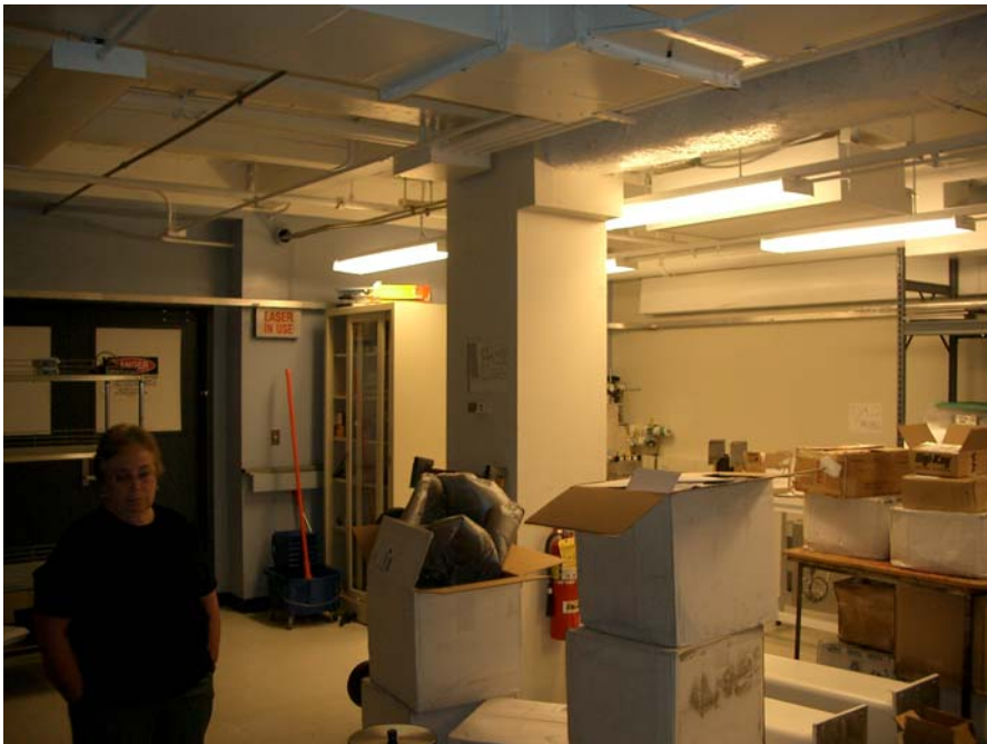
Figure 4 CO 2 Laser Lab Area (view line 'C-A' of Fig 1). Double doors to high bay on LHS of photo. Pillar across which laser curtain will hang at centre of photo.
