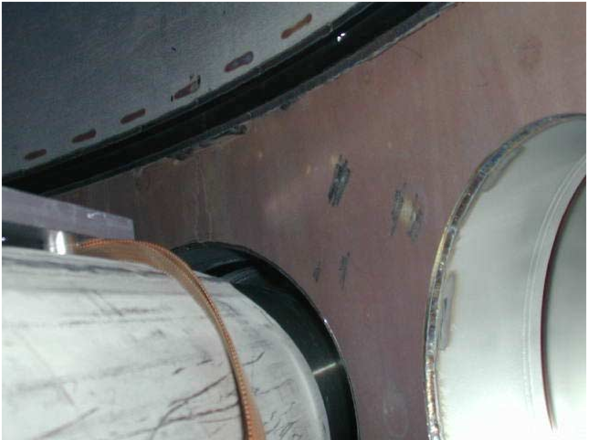
WBSC 8 May 12, 2000: 002. Cables tucked under NW corner, from N
