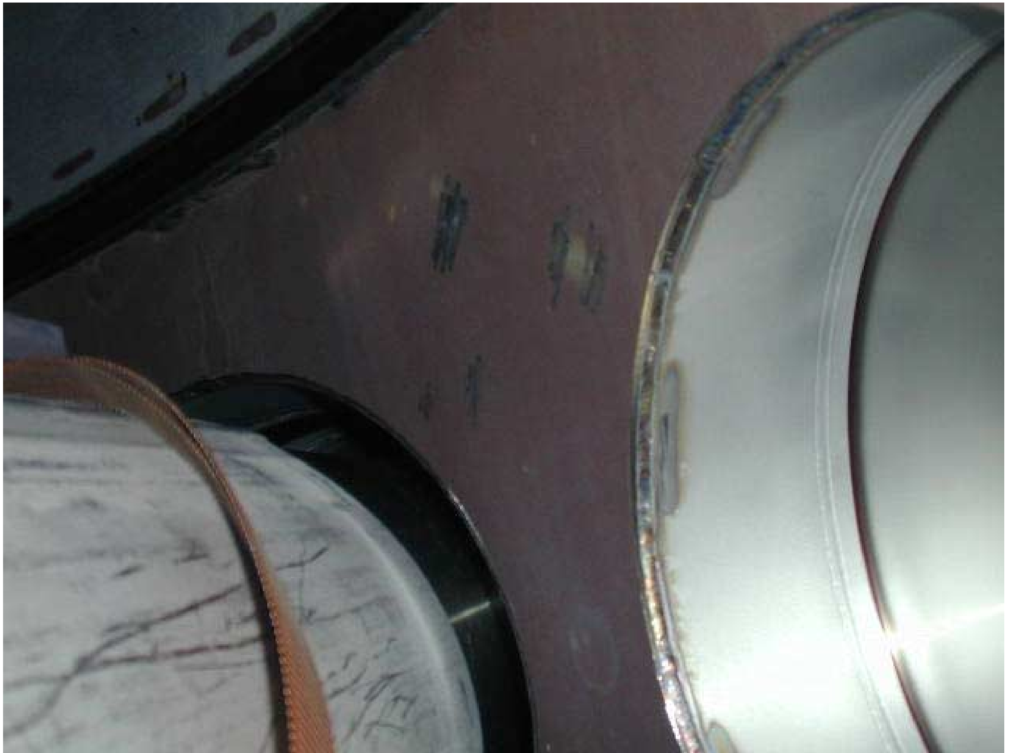
WBSC 8 May 12, 2000: 001. Cables tucked under NW corner, from N
