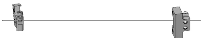
Fig 12: Upper Wire Assembly complete
